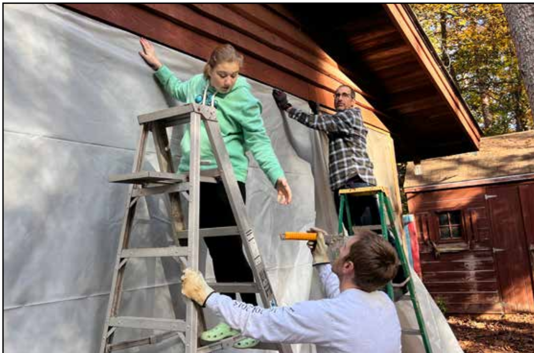
At their annual retreat, board members enjoy contributing to a project on the property. This year, attendees winterized the porches of Knoxwood Lodge by covering the screens with heavy plastic. This annual chore allows the porches to be used as additional gathering spaces during winter events. Pictured are Sam Pilc, Matthew Mahoney, and Will Kirk.
